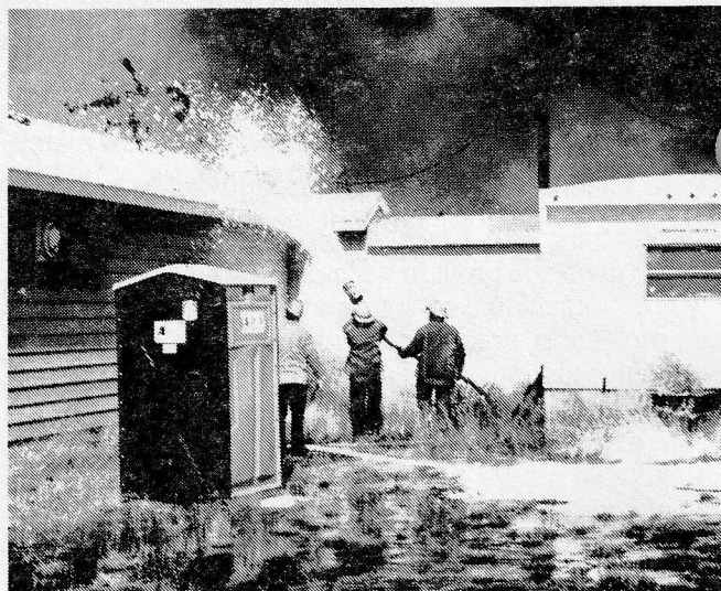
Figure 10. Single foam/retardant treatment may be preferable to this type of foam application repeated over several days.
